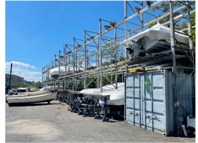
Rack Storage for 57 Boats
