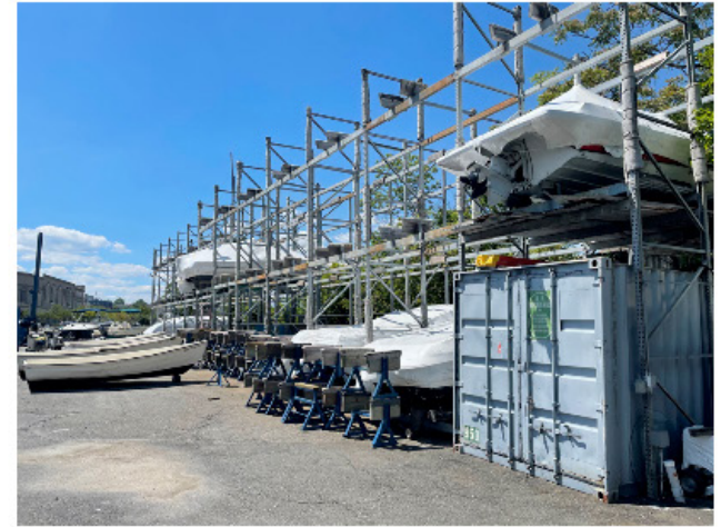
Rack Storage for 57 Boats
